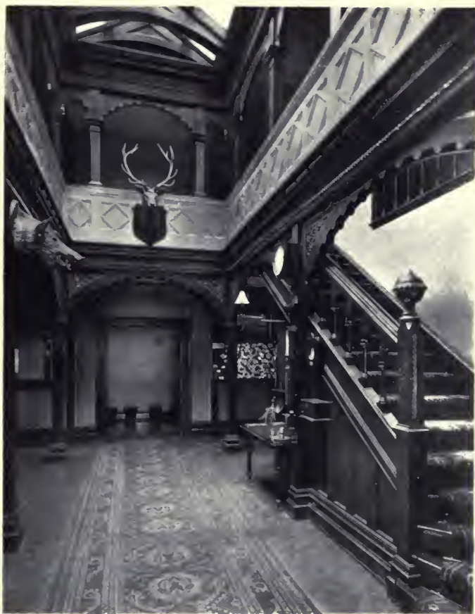
VESTIBULE. CHRISTCHURCH CLUB.
